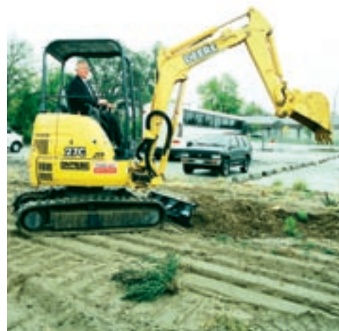
Breaking ground on the 3.7 acre site of Village Gate West – Sept. 26/05
