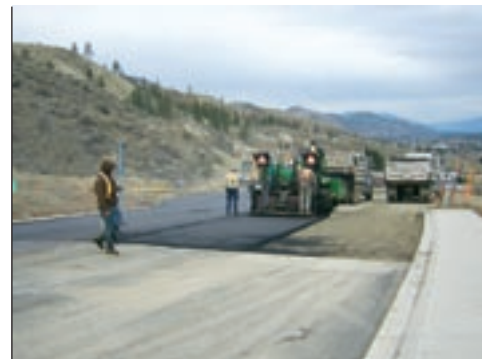
Street paving at Saddleback Hills – Phase I
