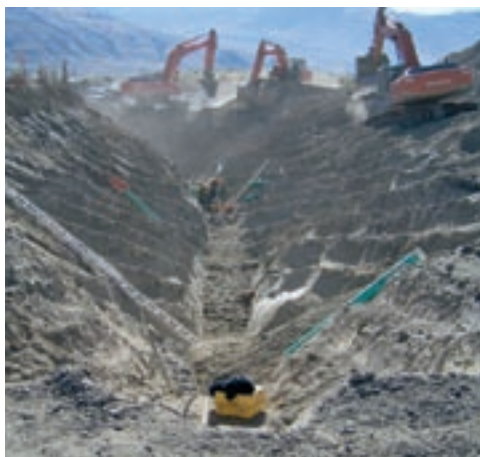
Extensive earthwork undertaken by Concert Properties, development manager for Saddleback Hills
