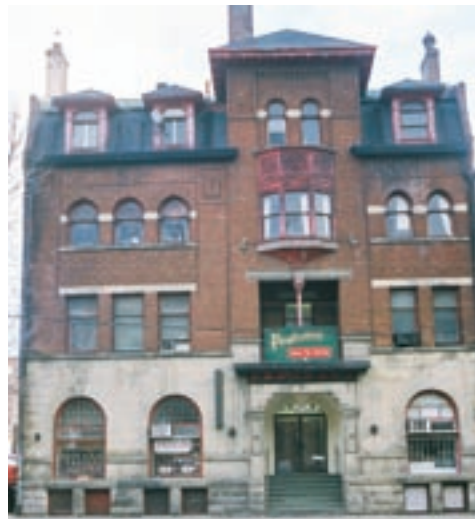
The heritage façade retained and integrated into Jazz on Church Street in Toronto
